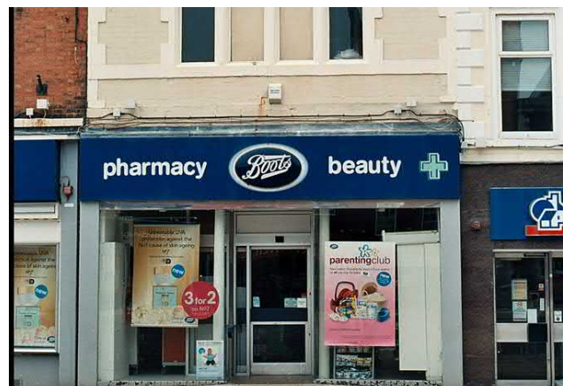
A poor example of a retail frontage where the shop front and branding have undermined the elevation of the host building
