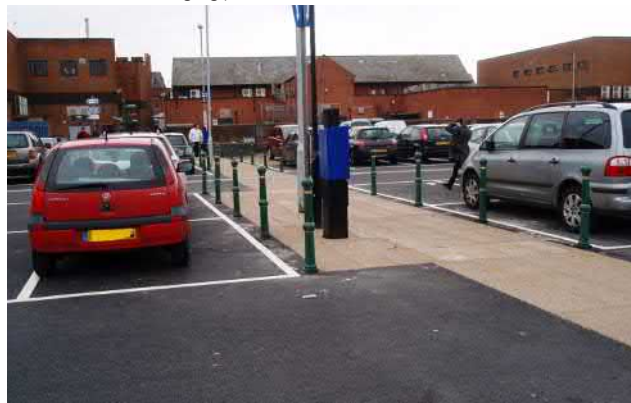
A poor example of a car park with no landscape features, electric charging points or cycle storage.
