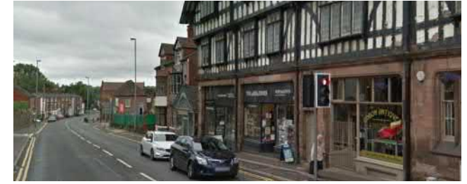
1. Long distance view from Broad Street
