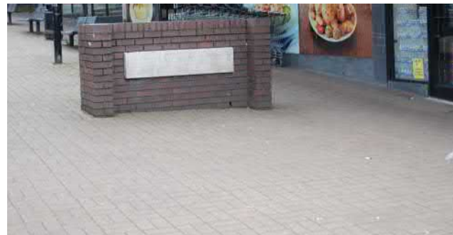
Basket weave pattern brick surfacing at the Smithfield Centre
