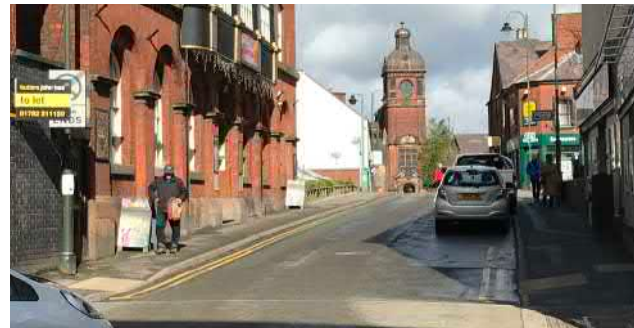
Tarmac paving along Market Street
