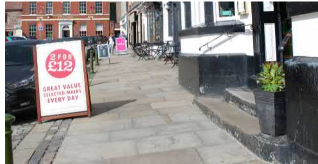
York stone flag paving around Market Place
